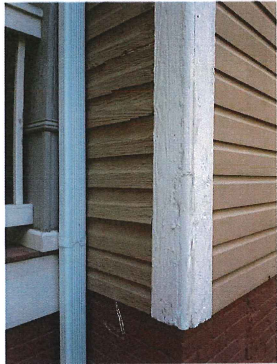
Original corner boards with 1/4 round
