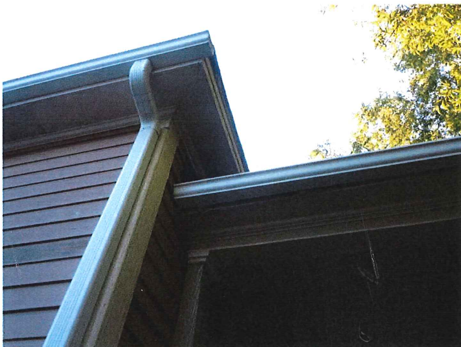
Front soffit detail at porch and house
